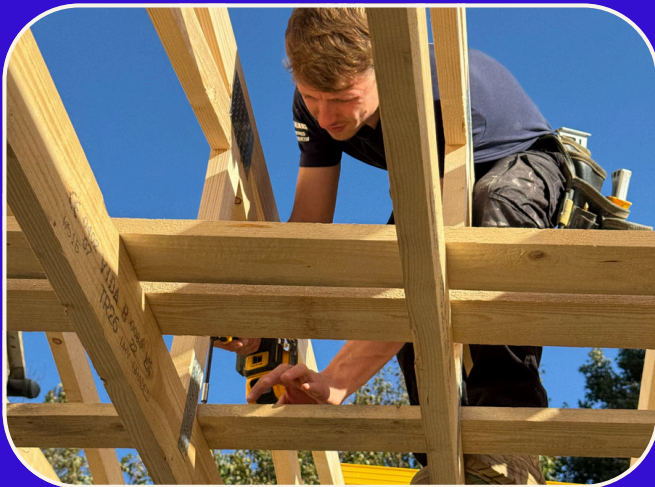
RESIDENTIAL EXTENSION PROGRESS
